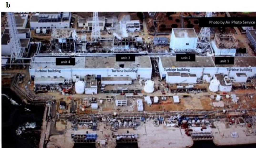
Figure 2. 1 (a) Hydrogen explosions and destruction of reactor buildings, panels (A and C) unit 1, panel D unit 2, panels (B and E) unit 3, and panel F unit 4 (b) Units 1, 2, 3, and 4 after the explosions [24].
